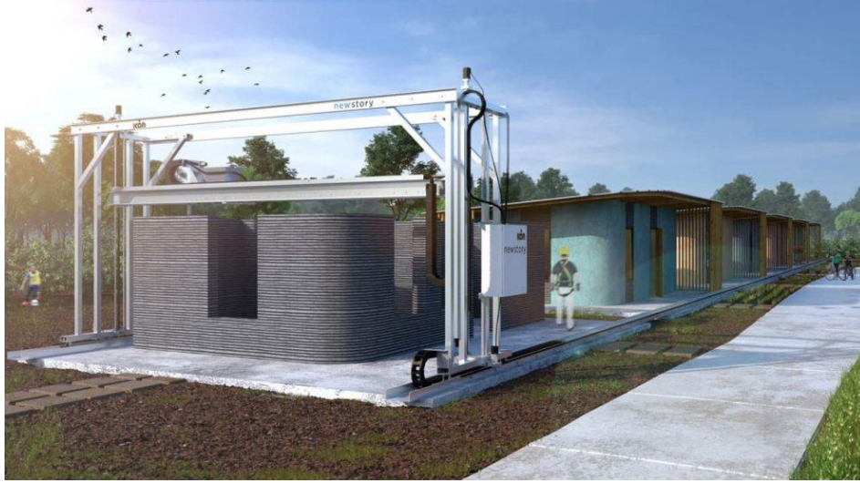
Şekil 9. Contour Crafting yönteminin şematik gösterimi (ICON Team, 2019) Figure 9. Visual representation of the Contour Crafting system (ICON Team, 2019)
