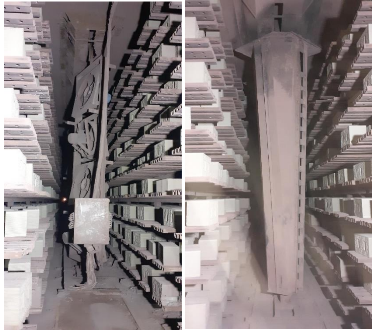
Figure 5. The axial and rotary fans in the dryer
