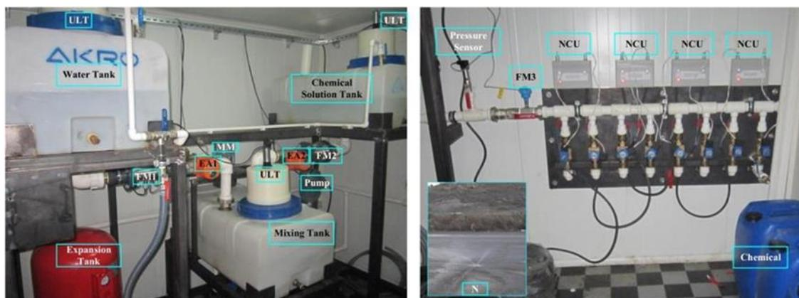
Figure 3. Implemented spray subsystem view
