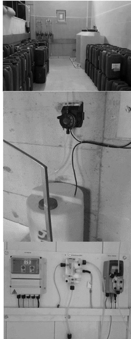
**Figure 3.** Drinking water sodium hypochlorite system
