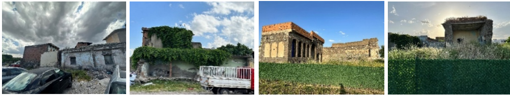
Figure 4: Buildings with minor and moderate damage
