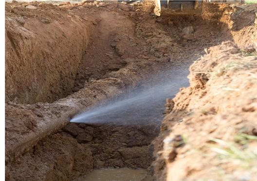
**Figure 4** Example images of underground faults causing physical losses in drinking water
