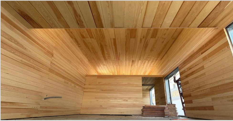
Figure 3. Interior and ceiling wall cladding made using wooden building materials
