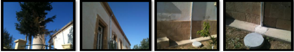
Fig. 9 a,b,c,d. Rainwater storage place in village mosque.
