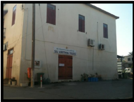
Fig. 12 a. Water Treatment Plant.
