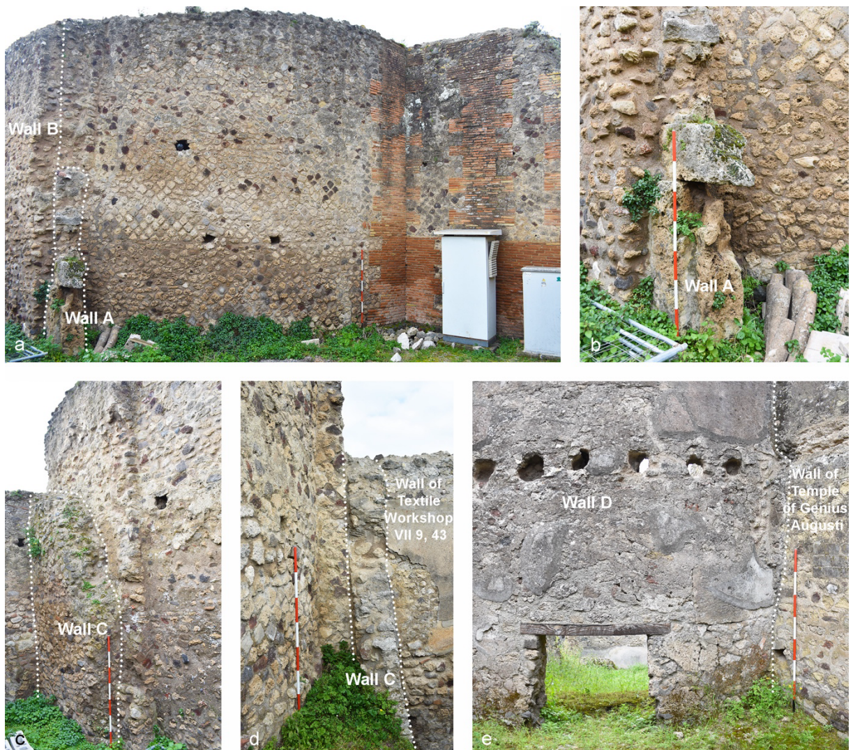
Fig. 6. Sanctuary of the Public Lares: earlier structures incorporated in the building: a, b) limestone ashlar wall A with the reinforcing wall B; c, d) plastered wall C; e) wall D and the junction with the Temple of the Genius Augusti
